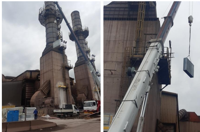
Above and Right: Design and placement of the silencer
